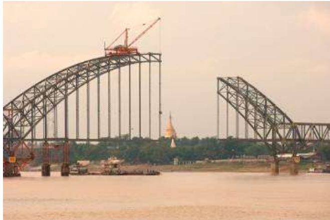
Bridge being constructed over the Irrawaddy River
